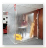
Plastic sheeting is used to outline the proposed work-zone and cover windows. These barriers are used to prevent the spread of mold to unaffected areas of the residence during the demolition portion of our work and to prevent infiltration of outside air into our work-zone.
